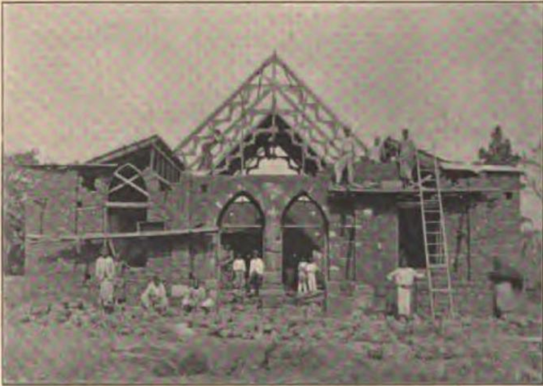
NEW MISSION CHAPEL IN BUILDING, SAN SALVADOR
