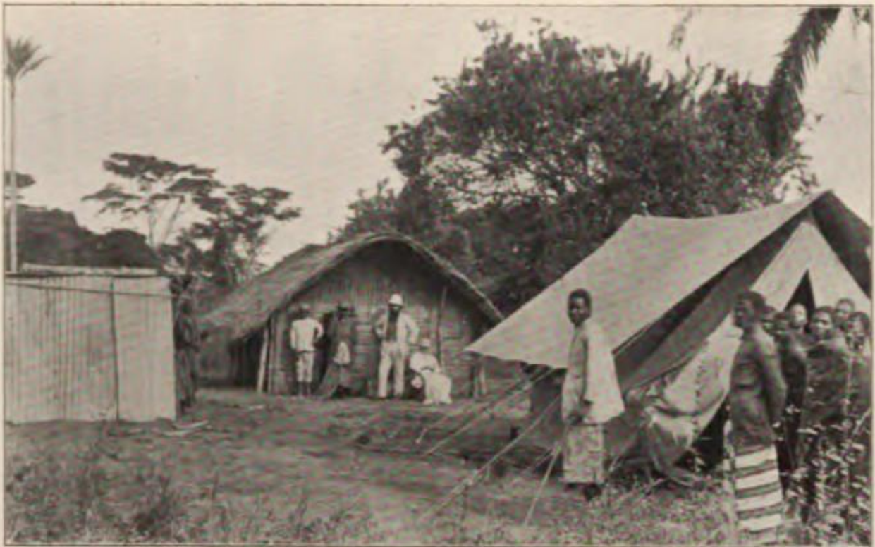
COMMENCING THE NEW STATION AT KIBOKOLO, ZOMBO
